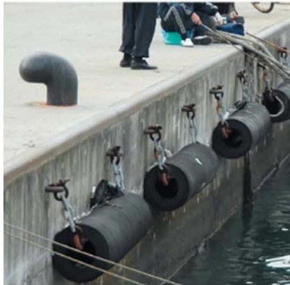
Gambar 6. Rubber fender silinder
