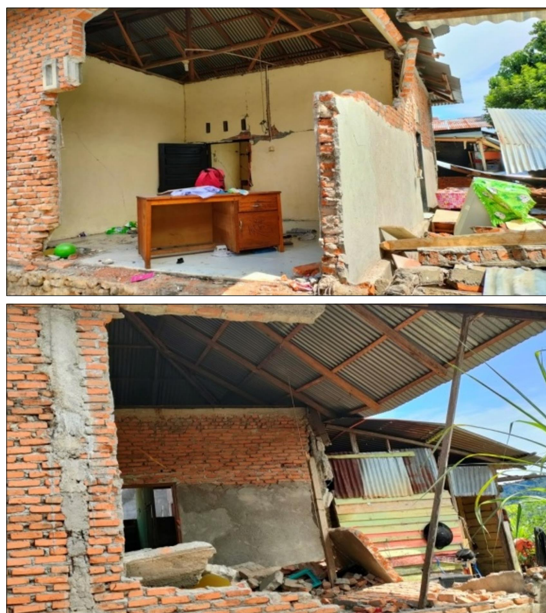
Figure 6. Damage to columns, walls cracked and collapsed
