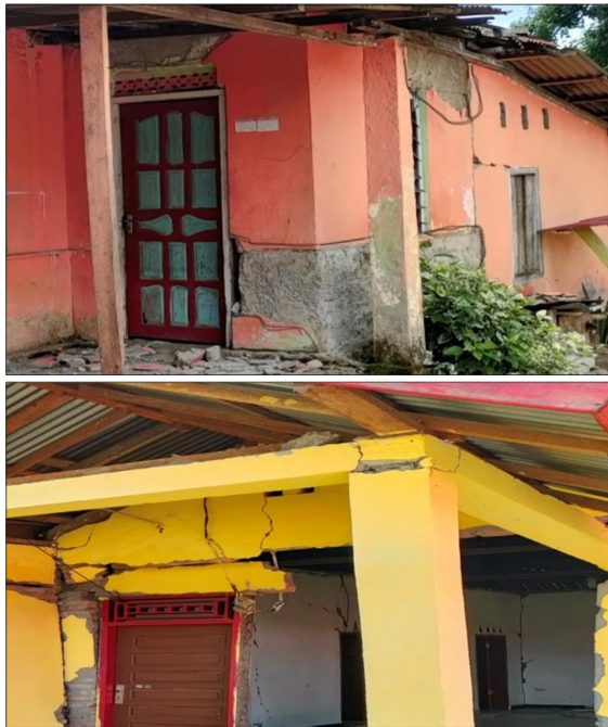
Figure 5. Damage to walls and column structures
